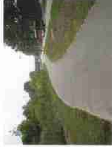
Figure 8: Slope on hard surfaces direct surface run-off through green areas (NC State University campus).
