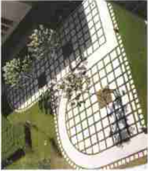
Figure 4: Design should encourage the use of porous material on large lots and roads.
