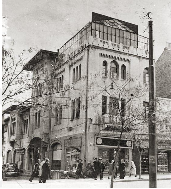
F. 170. (solda) Halk Bank Binası, 1949 (Kaynak: https://www.facebook.com/photo.php?fbid=221963185855390&set=gm.2904735136236248&type=3&theater&ifg=1 )
